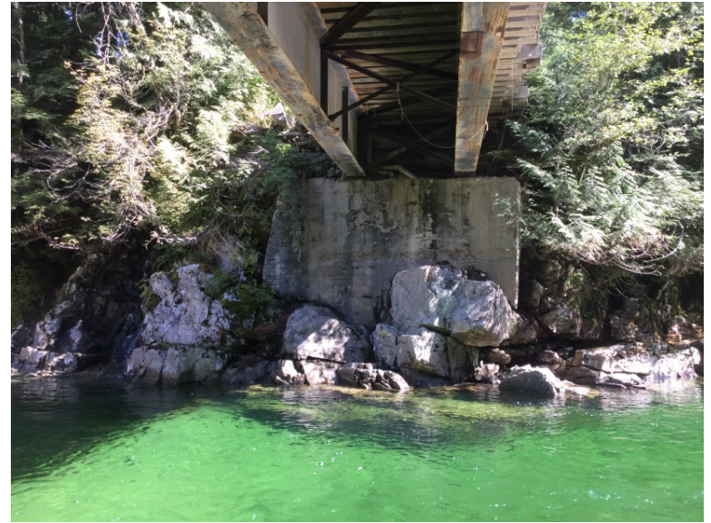
Left Bank Abutment when facing downstream
