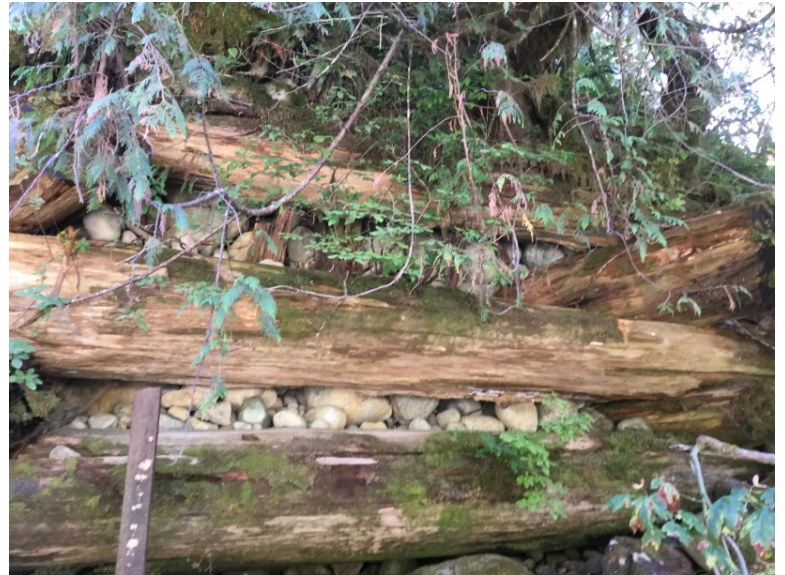
Upstream right bank wingwall condition
