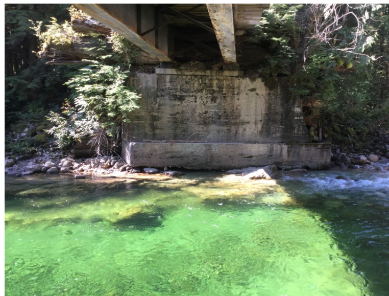
Right Bank Abutment when facing downstream
